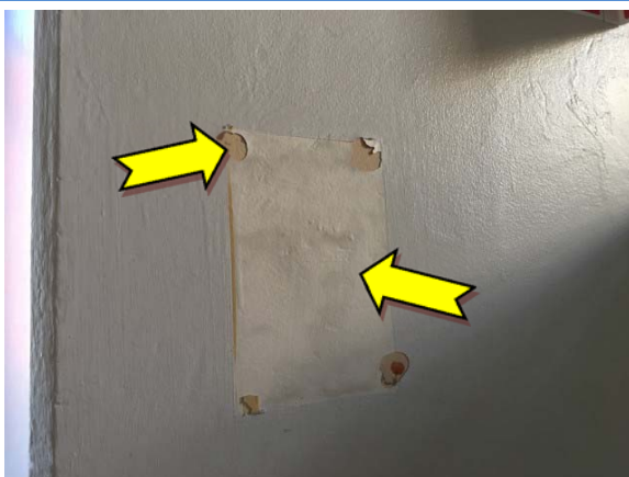
Photo 11. Interior, ground level, hall, throughout, walls – suspected lead-containing yellow and white lower coloured paint systems.
