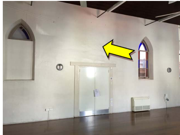
Photo 10. Interior, ground level, hall, throughout, walls – suspected lead-containing cream upper coloured paint system.
